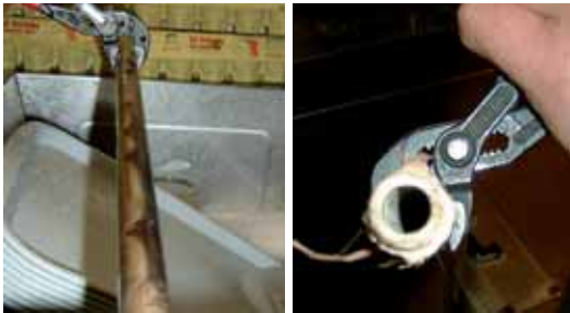
The nozzle fitting without limescale deposits. The nozzle holes are absolutely clear.
